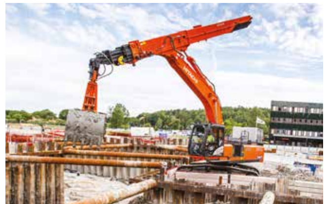
Special application excavators
