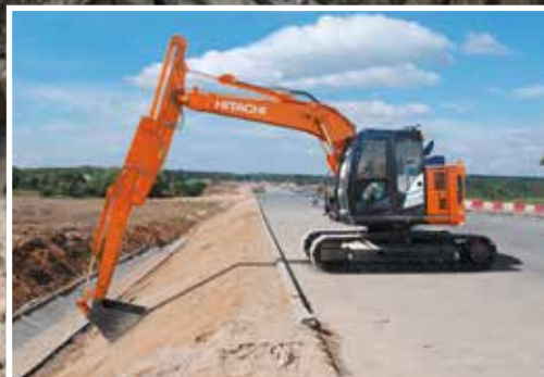
Combined operation of boom and arm enables smooth slope finishing.
